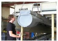
Mount Front Trim Plate between front cross channel and Toon-Trac and install back angle stop. Move Bow Eye to top of Front Trim Plate if under deck.
